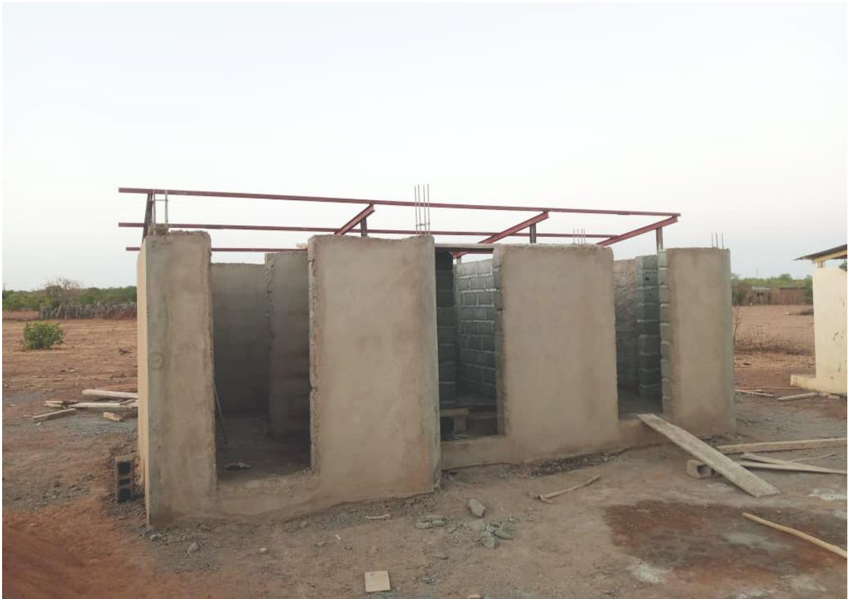
Front side, plastering in progress
