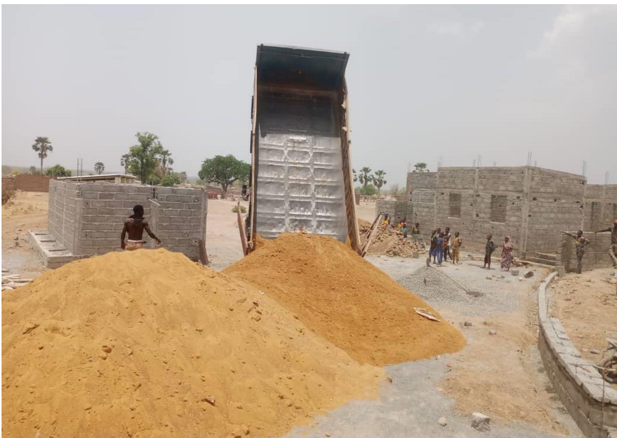
Filling material for the pedestal. The soil will be later compacted and covered
