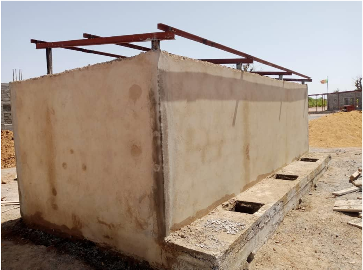
Back side, plastering in progress
