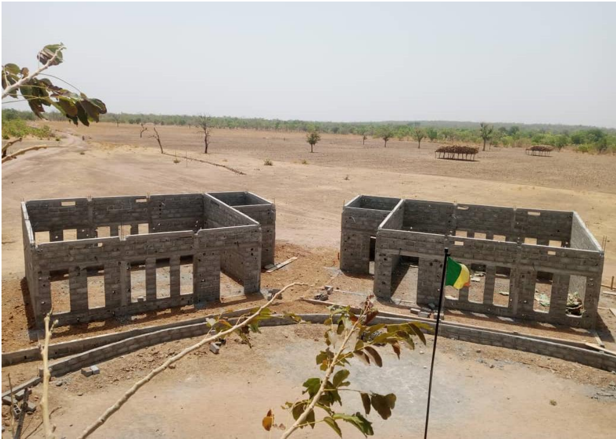
View of the classrooms. The perimeter structure of the pedestal is completed
